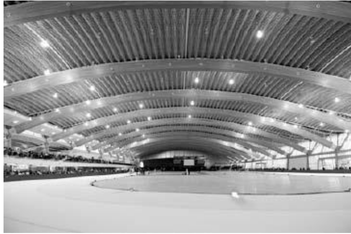
The interior roof of the speed-skating arena for the Vancouver 2010 Winter Olympics was made entirely of engineered wood.
